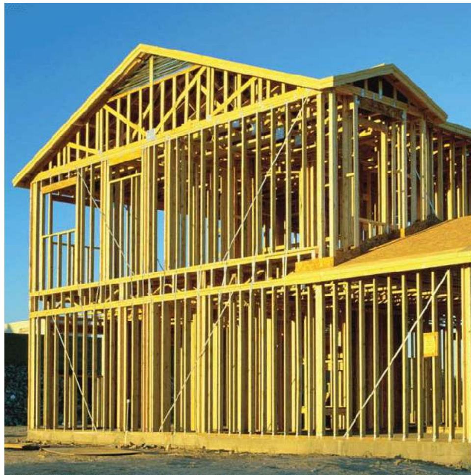
2015: Typical Wood Frame Structure
