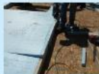
Adjust the height of the circular saw blade to protect the framing.
