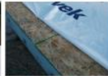
Staple WRB into place. Fold back and tack long edges that need to wrap down or around when the wall is later ripped up.
