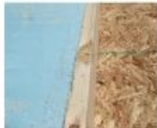
Adjust the height of the circular saw blade to protect the framing.
