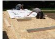
Attach WRB before wall erection to save time and effort. Use cap nails or wide staples.
