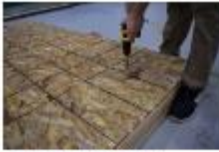
Snap chalk lines and drill holes.
