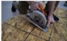
Seek the circular saw to catch the first drill hole. Do not overcut at corners.
