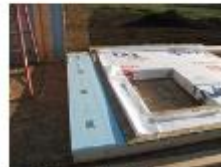
Two adjacent sections of wall must be planned to stagger the vertical joints of the rigid foam and OSB.
