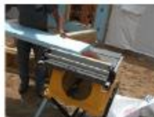
A table saw trims 2-in. rigid foam cleanly, with little waste or debris.
