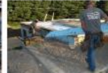
Tack c.i. rigid foam to rim band.
