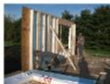
Two adjacent sections of wall must be planned to stagger the vertical joints of the rigid foam and OSB.
