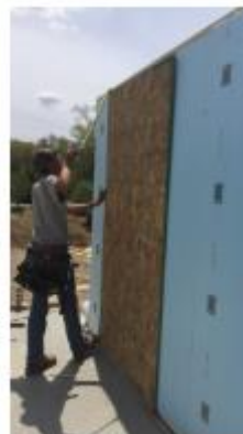
One sheathing must always be oriented vertically, for structural bracing.
