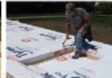
Cut window openings for window installation and detailing guidance on page 20.
