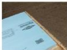
Measure and cut rigid foam for a snug fit between the EP&B wall's top and bottom plates.
