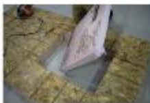
Remove the foam from the opening.
