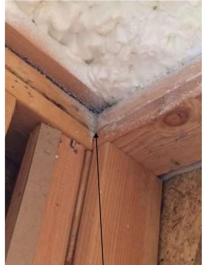
Seal formed at corner of wall assembly
