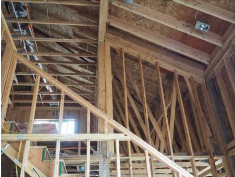
Exposed roof deck
