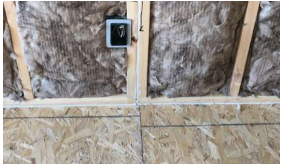
Caulk at sill plate
