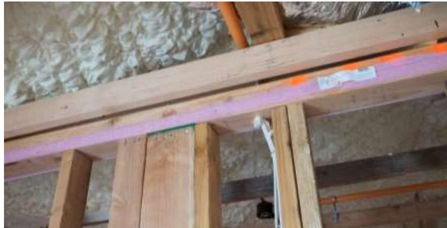
Foam gasket to seal drywall to top plate
