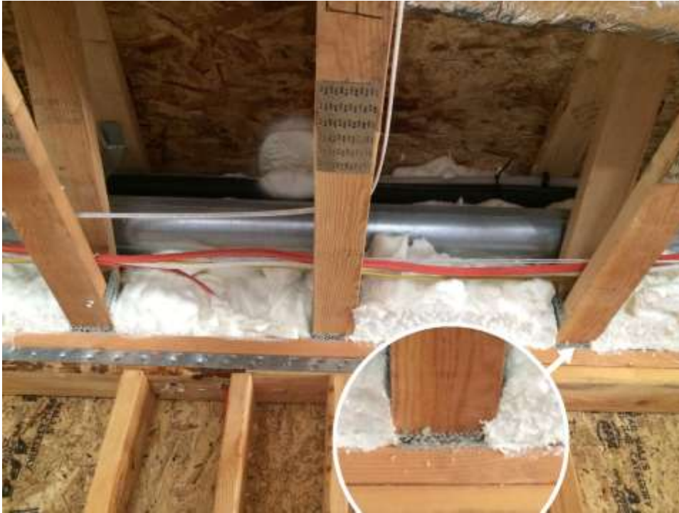
Seals formed under trusses
