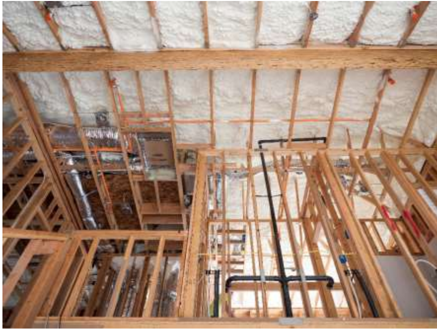
Foam at roof deck
