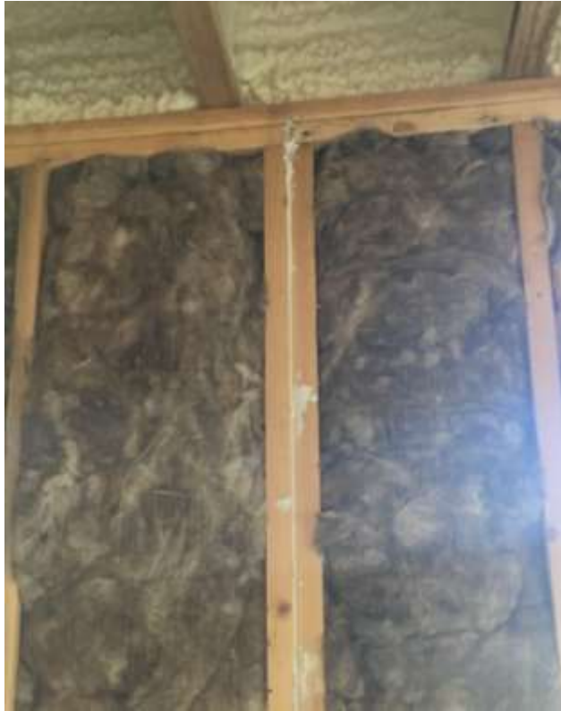
Caulk at seams where wood is joined
