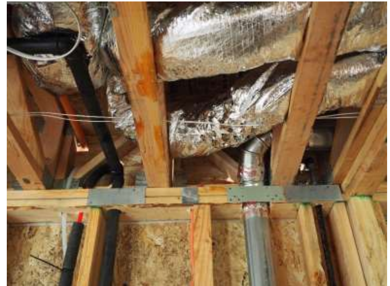
Rim joist penetrations
