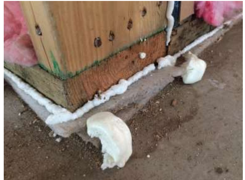
Can foam and gasket at sill plate
