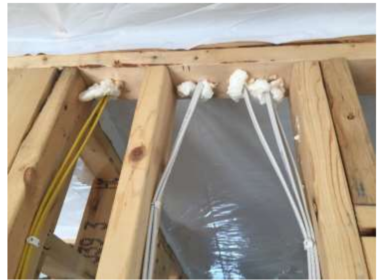
Can foam at wire penetrations
