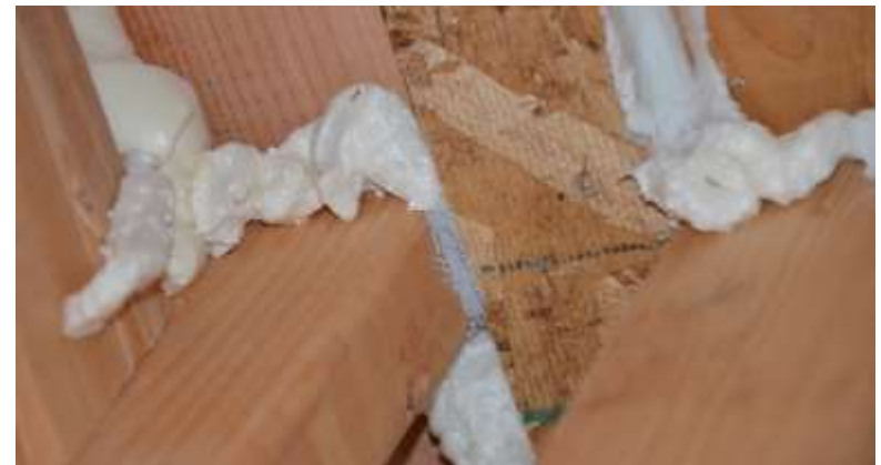
Seal formed between gap in foam
