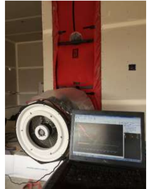
Blower door setup for pressurization
