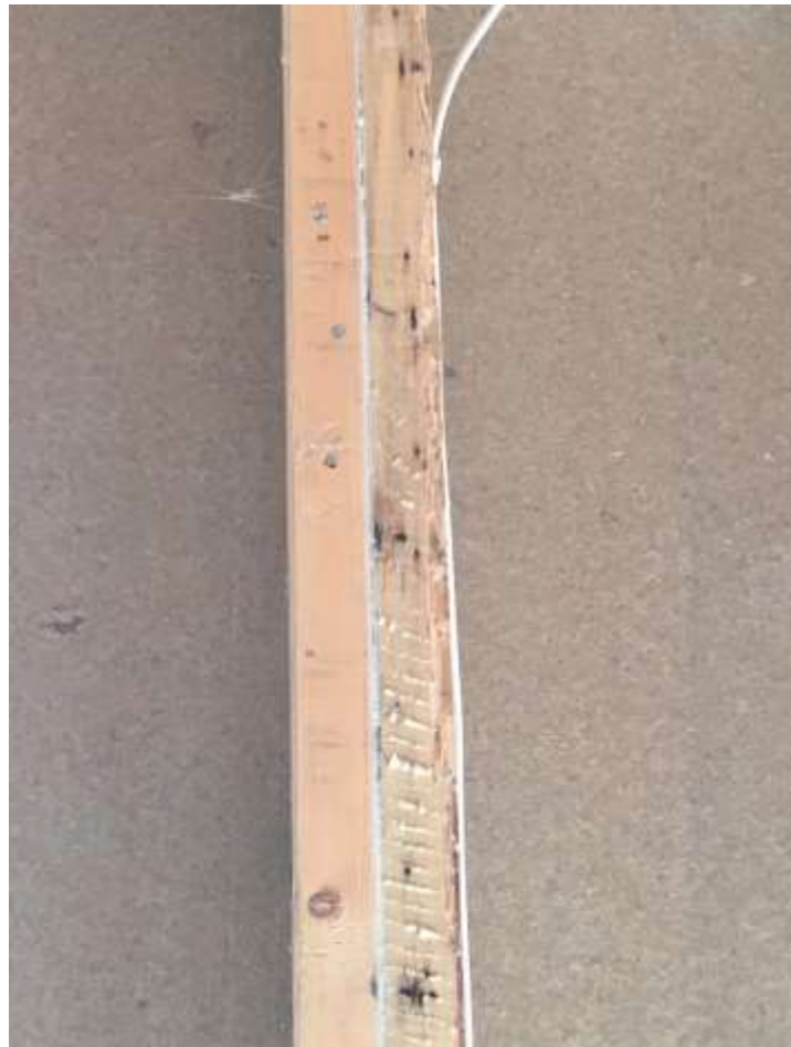
Seal formed between studs
